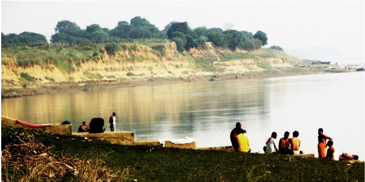
Image 44 : Erosion Prone Bank At Chaturmukh Ghat
